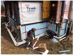
Narthex - seismic upgrade to stiffen front end of building and strengthen organ loft.
